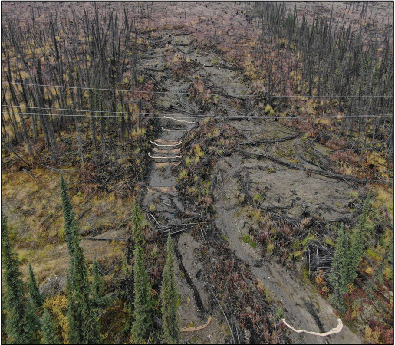
Figure 2. Aerial Shot of Completed Erosion Control Installation
