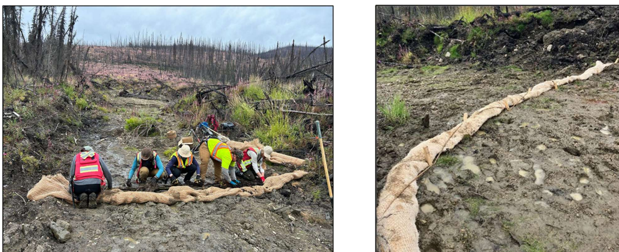
Figures 5 & 6. Non-Live Materials: Team installing Erosion Fabric and installed Sediment Log
